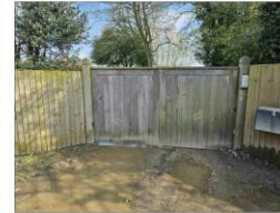
EXISTING SOTHERN ENTRANCE
